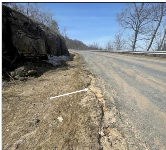
Figure 14. Arrow pointing to possible Prairie Du Chien Gp/Jordan Fm. contact in ditch just below road grade.
