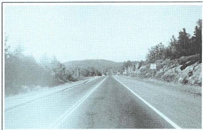
A sight-hidden dip on Highway 11-17 near Thunder Bay
