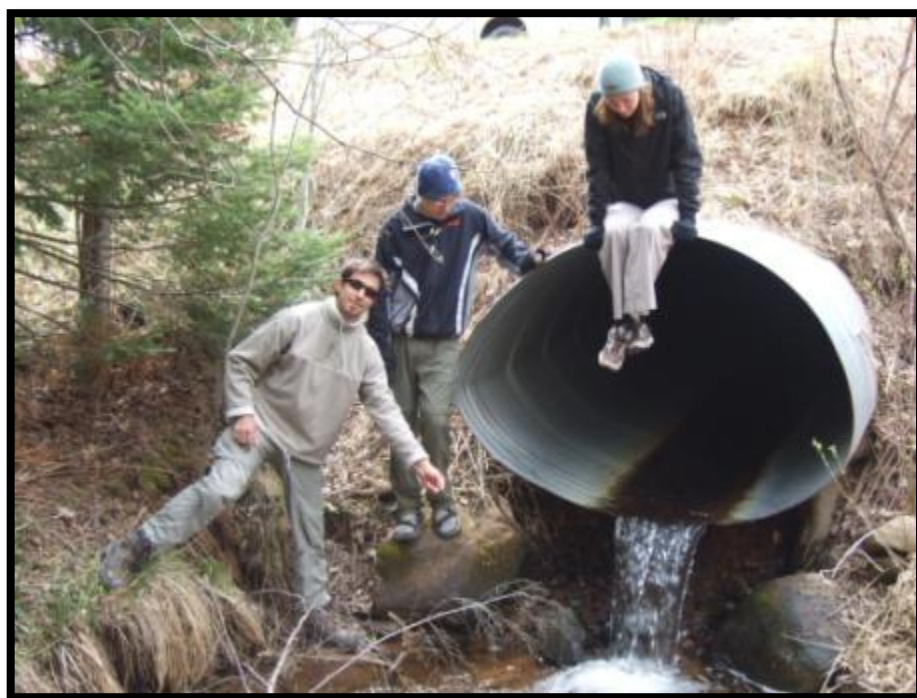
Hagger Road west culvert – before replacement. -T. Fitz
