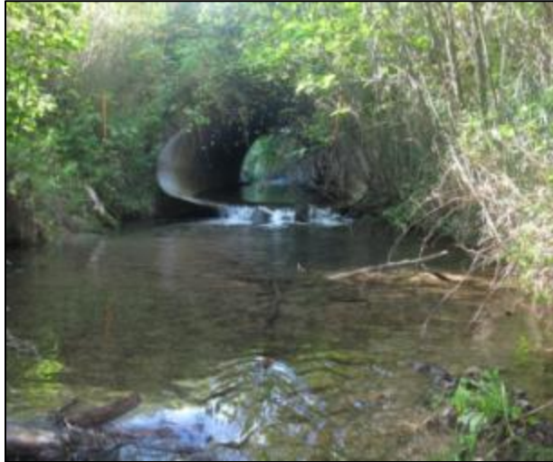
Figure 7. Culvert at Troutmere Creek.
