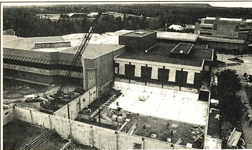
Construction of the Student Centre and Regional Education Centre is progressing right on schedule for completion in September 1991.
