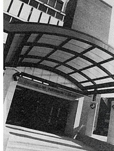
Lakehead has just completed extensive renovations to The Chancellor Paterson Library
