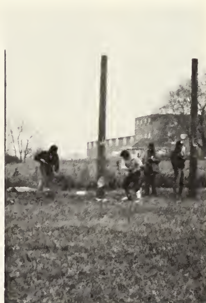
Felling hydro poles.
