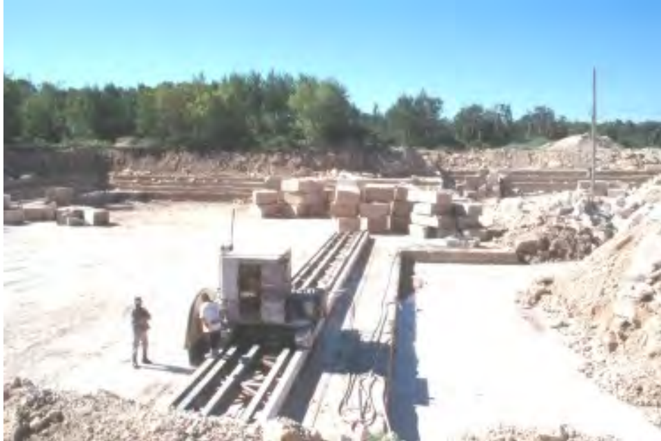
Figure 12. Carbide toothed circular saw in Gillis Tyndall Stone Quarry.
