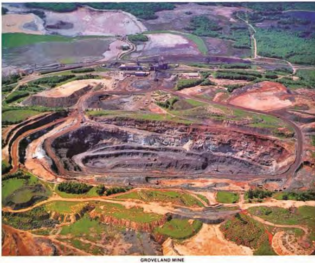
Figure 6. The Groveland Mine has a long history that began in the late 1880's and continued into the 1980's. This view, probably from the 1970's, is looking south with the plant in the upper central part of the air photo. Source M. A. Hanna Company. Archives of the Michigan Department of Environmental Quality.
