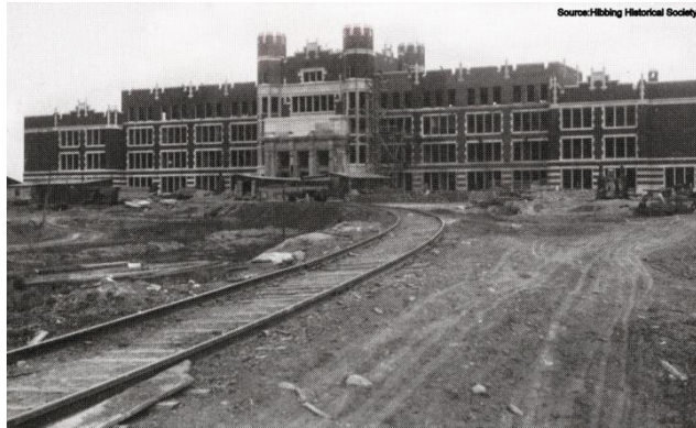
Figure 7- Hibbing High School under construction.
