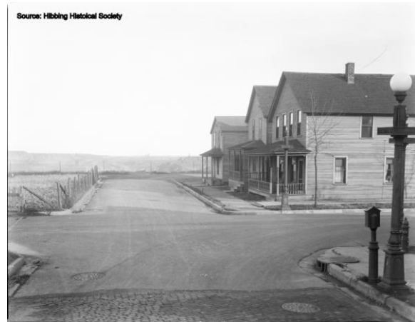
Figure 13- North Hibbing at crest of Mining.
